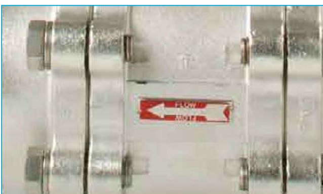
Indicator on valve body
